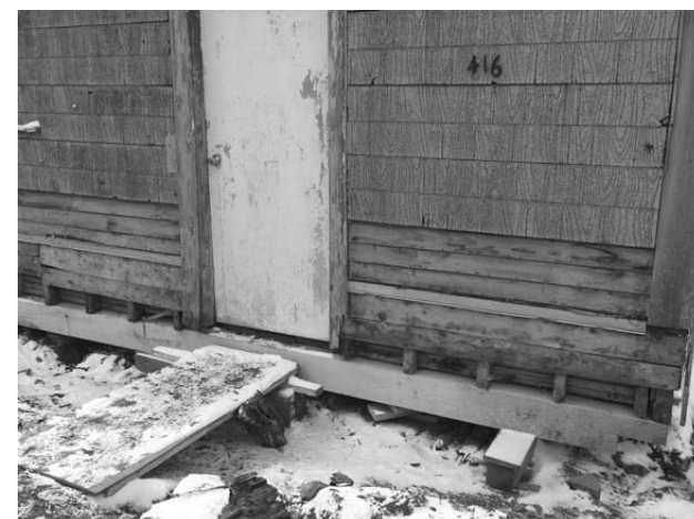
Mohawk Grange of Colebrook gets some much-needed repairs.
